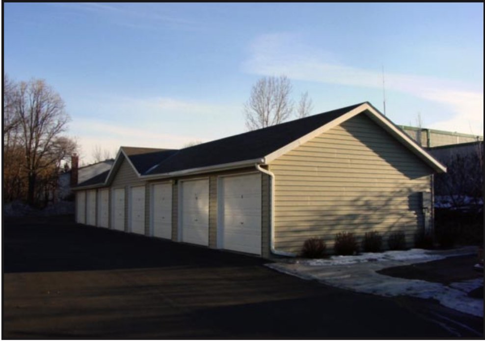
VIEW OF DETACHED GARAGE BUILDING
