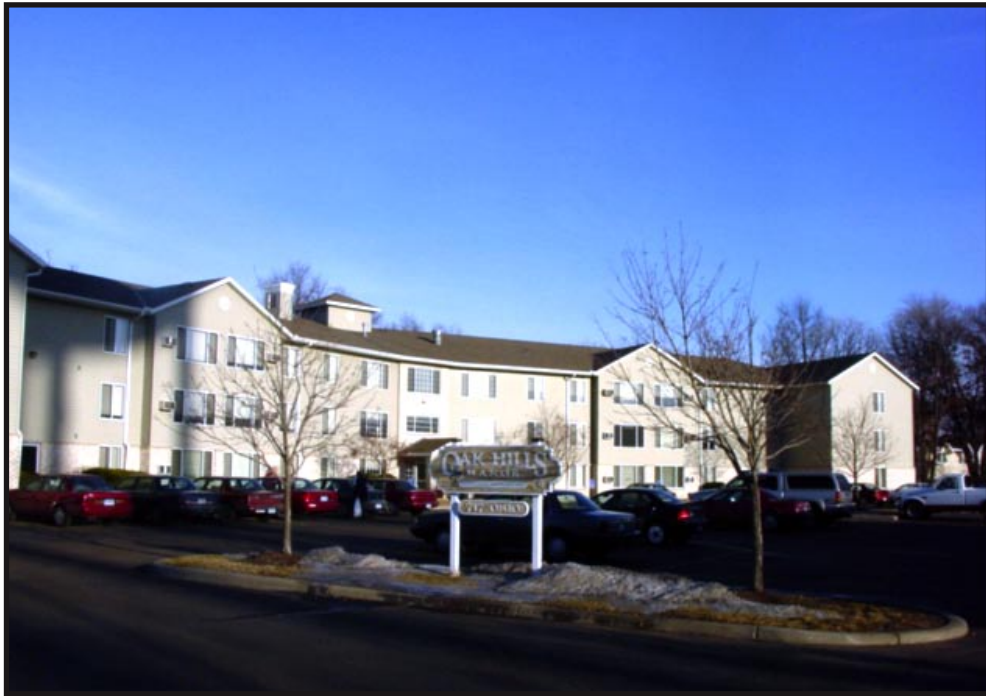
VIEW LOOKING EAST FROM CIVIC HEIGHTS DRIVE
