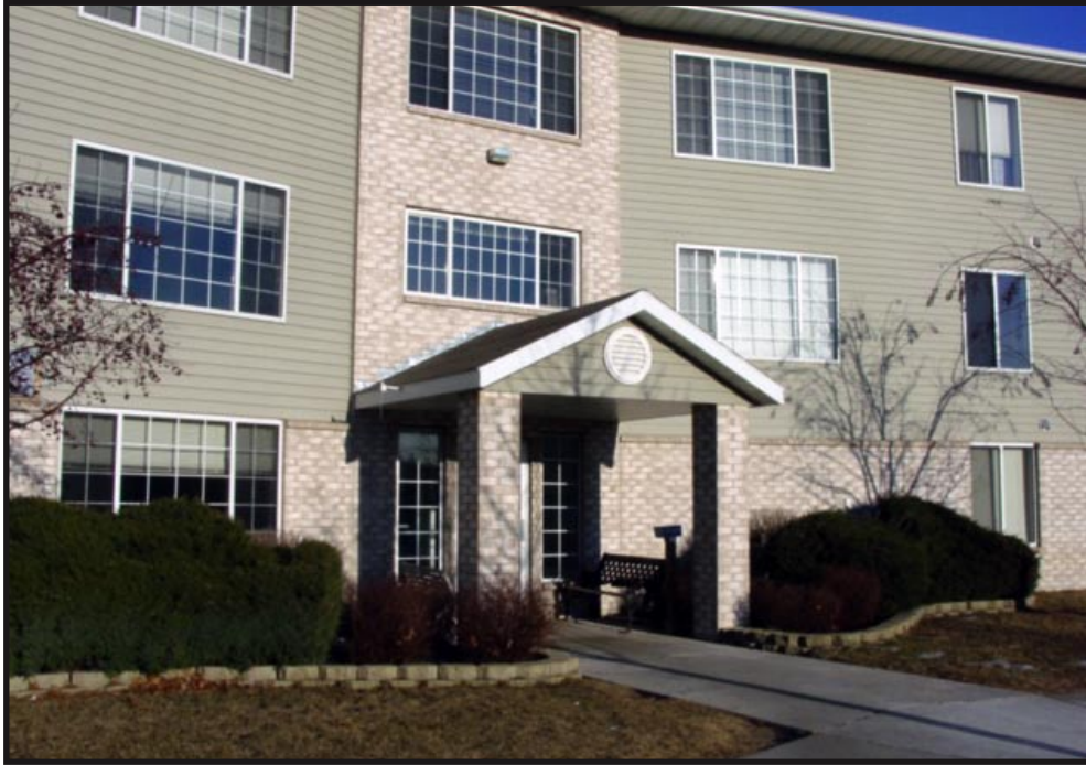
VIEW OF FRONT OF BUILDING
